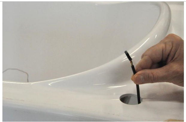
Pull keypad cord through hole.
