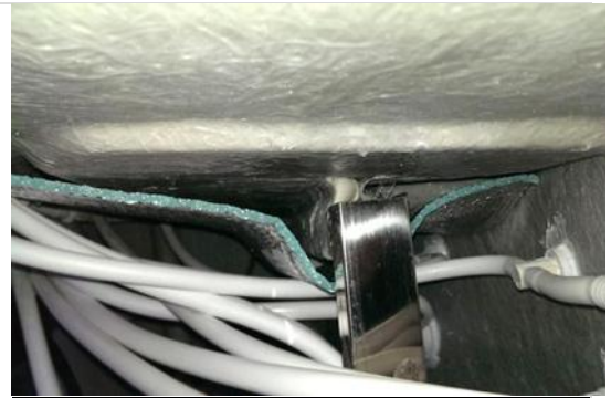
Wrap heater over tub frame if needed.
