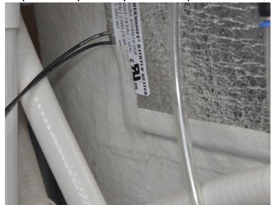
Optional - place tape around perimeter.
