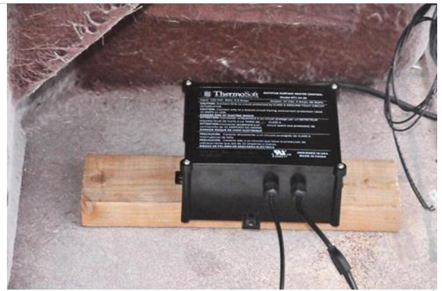
Or, mount control 1.5" above the intended tub/shower mounting surface (finished floor).
