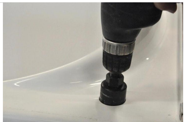
Drill 1.5" (38mm) hole in tub; clean dust from surface & wipe with alcohol.
