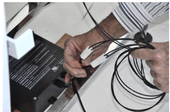
Connect heater(s) to control.
