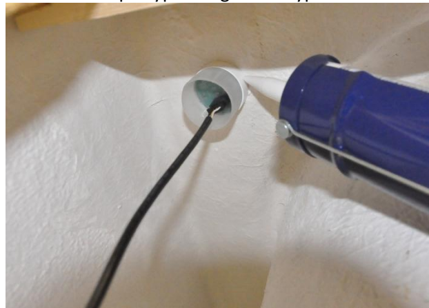
Apply silicone seal around underside of keypad.
